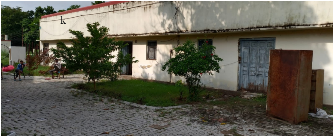
Mechanical Maintenance Section Building
