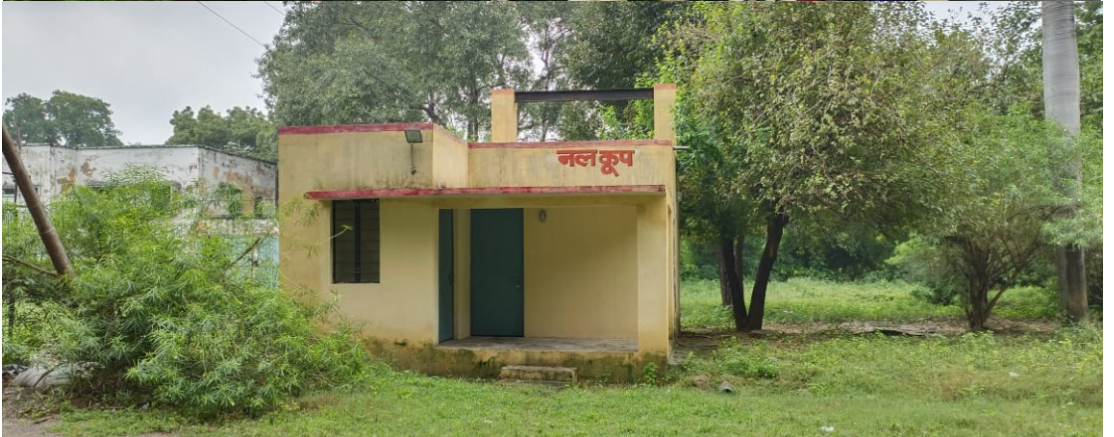
Overhead Water Tank & Pump House in the East Campus
