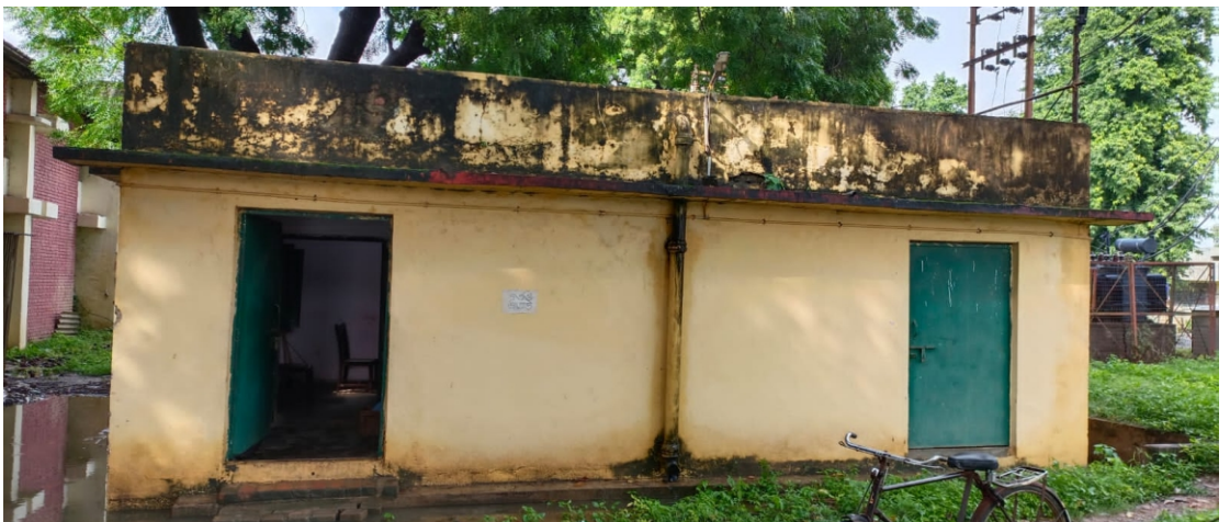
Electrical Maintenance Section Office
