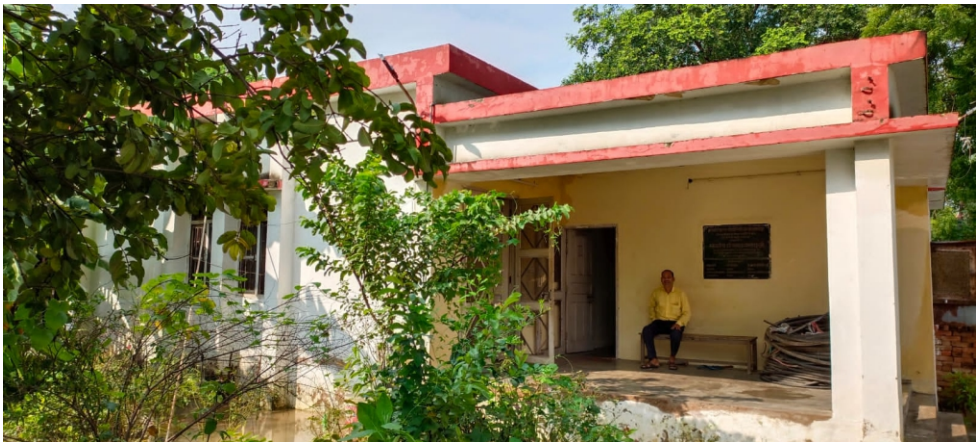
Office building of Electrical Sub-station
